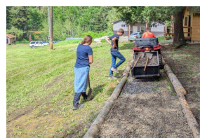
WORK ON NEW TRAIL BETWEEN CABINS
